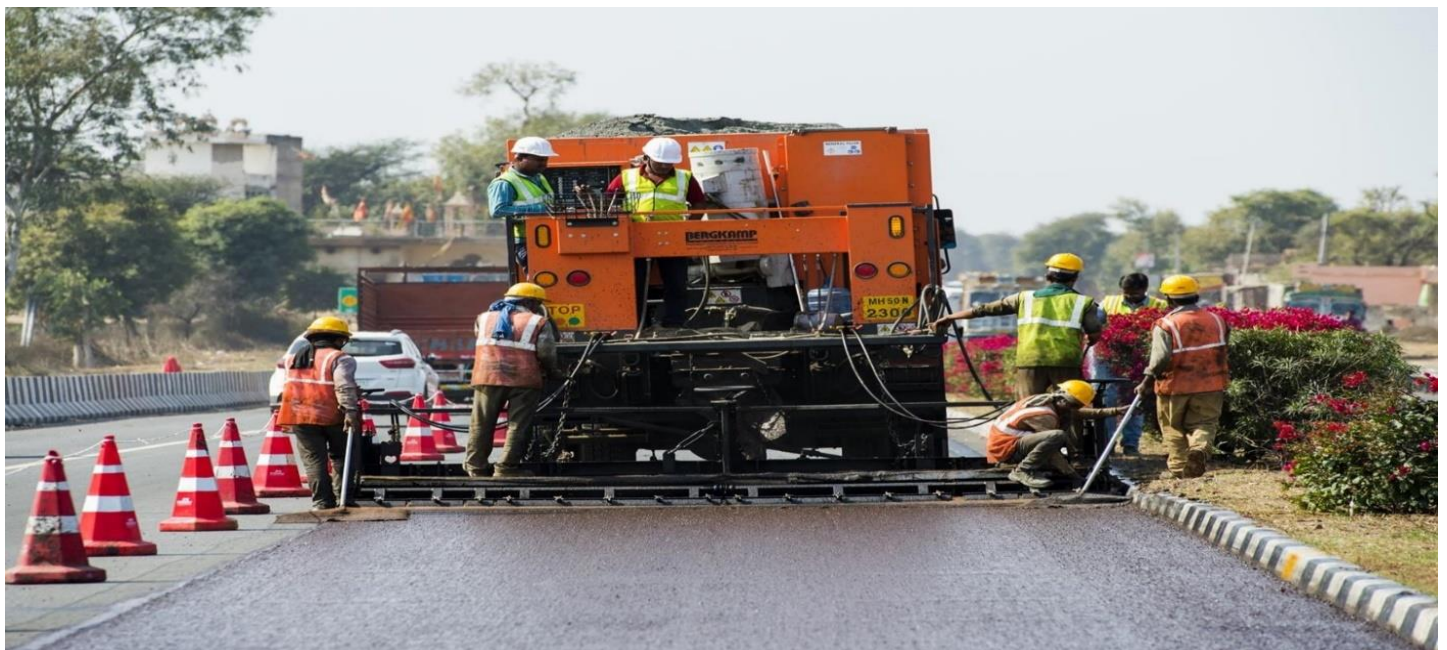
Figure 7. Microsurfacing
